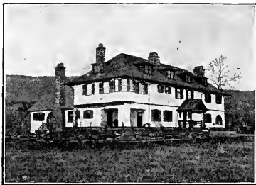
Residence of Thomas Shields Clarke, Esq., Lenox. Stained with Cabot's Shingle Stains and lined with Cabot's Sheathing Quilt for warmth. Wilson Eyre, Architect, Philadelphia.
